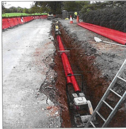
Image 5: Typical 38kV Underground Duct Installation
